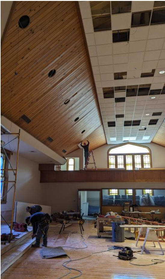
The sanctuary remodel is progressing! Lights are going in, steps for the platform are being re-constructed, the drywall is in, and mudding and taping is getting done!
